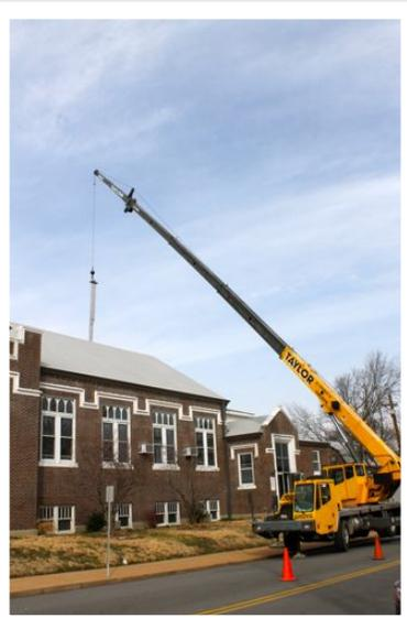
**Flue liner being dropped in place - one more step for our heating system.**
