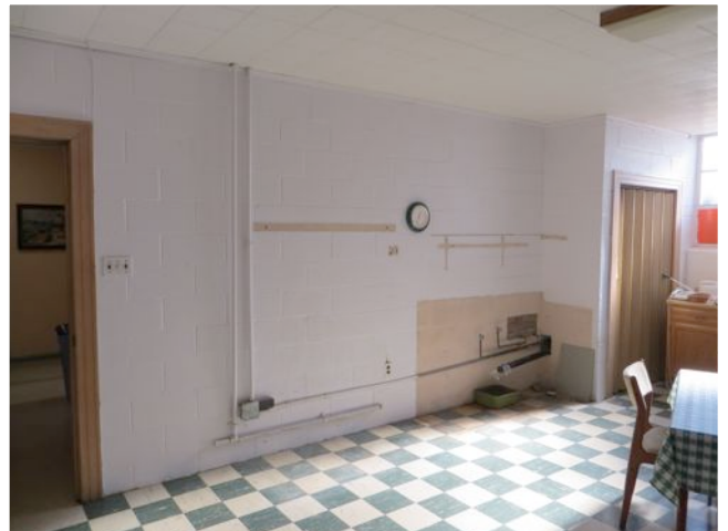
Kitchen area cleared out
